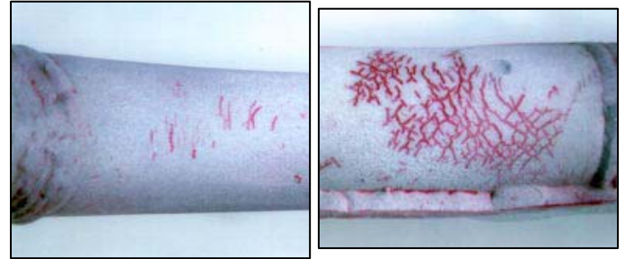
Figure 4: Dye-marked circumferential and crazed tube cracking
