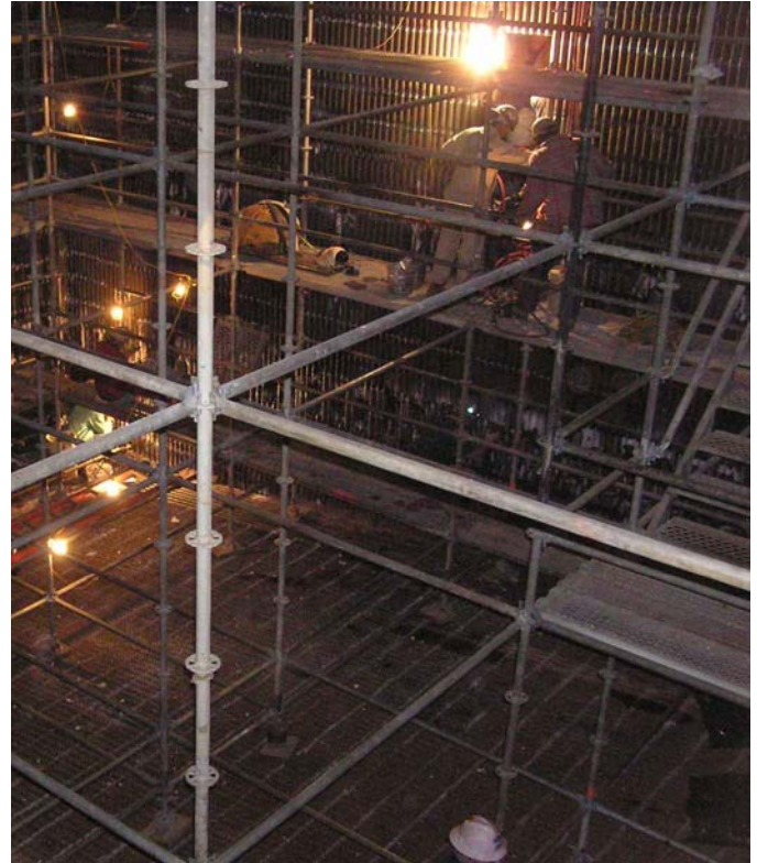
Figure 6: Interior view of recovery boiler during tube maintenance and replacement
