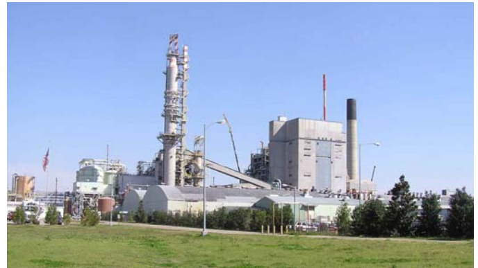
Figure 1: Recovery Boilers are the heart of the pulp and paper making process, and the largest single structure at a mill
